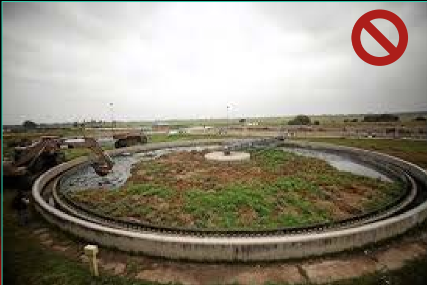
A: Sabokeng WWTW, Emfuleni (2019)
